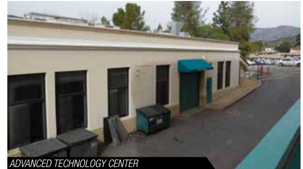
ADVANCED TECHNOLOGY CENTER
