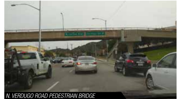
N. VERDUGO ROAD PEDESTRIAN BRIDGE
