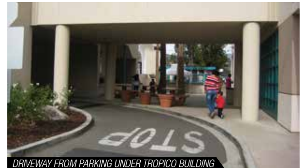
DRIVEWAY FROM PARKING UNDER TROPICO BUILDING
