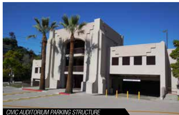
CIVIC AUDITORIUM PARKING STRUCTURE
